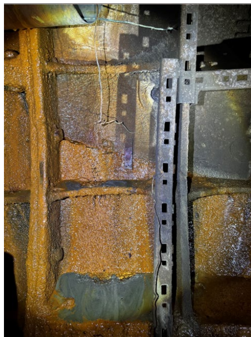
Fig. 4. Leaching and wet spot in the inter-ring and inter-block joint of the lining, active leak. A crack in the back of the tubing
