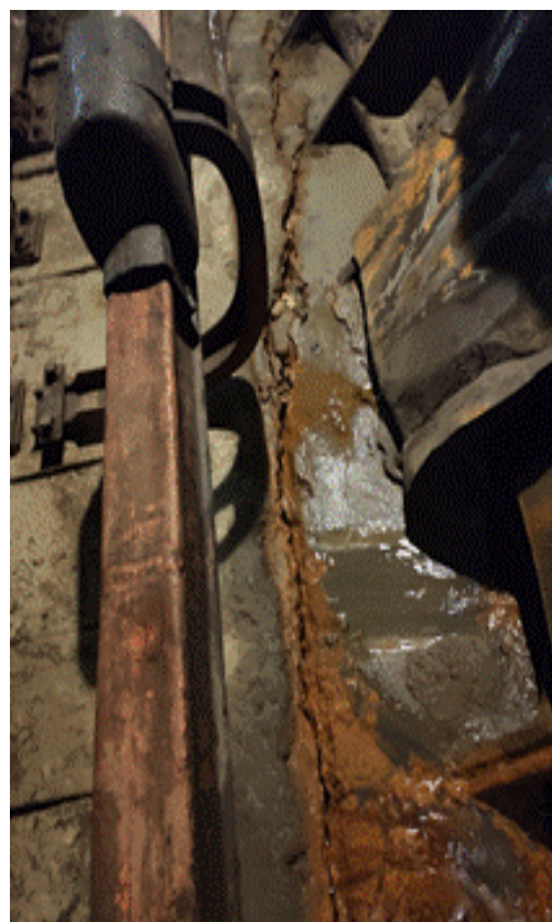
Fig. 2. Soil washout into the area of the contact rail
