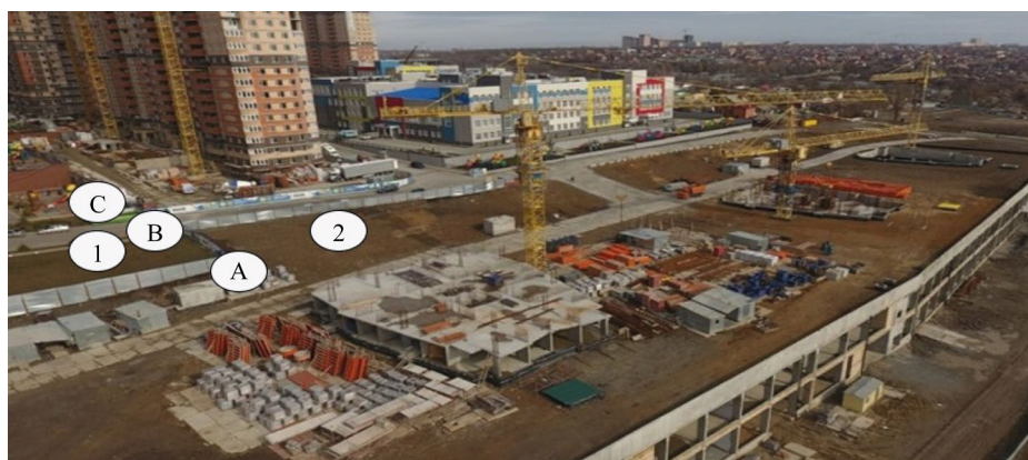
Fig. 2. Construction site of an infill development: 1, 2 — planting sites; A, B, C — control points for measuring the PM 10 concentration
