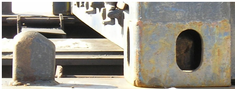
Fig. 7. Stationary stop for the container
