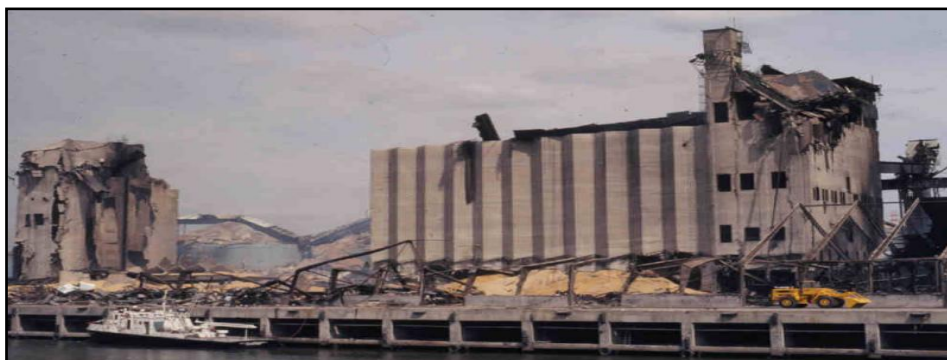
Fig. 1. Explosion of dust-air mixture in elevator grain storage sections
